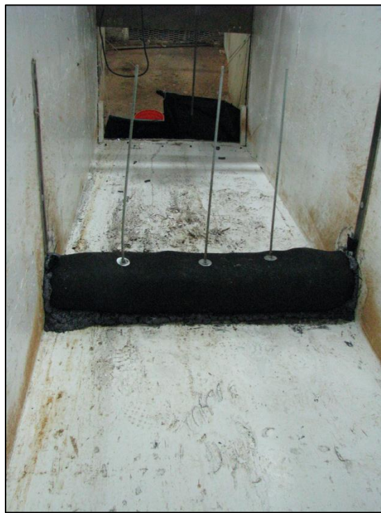
Figure 2-4. Photograph of 12-inch E-tube installation
